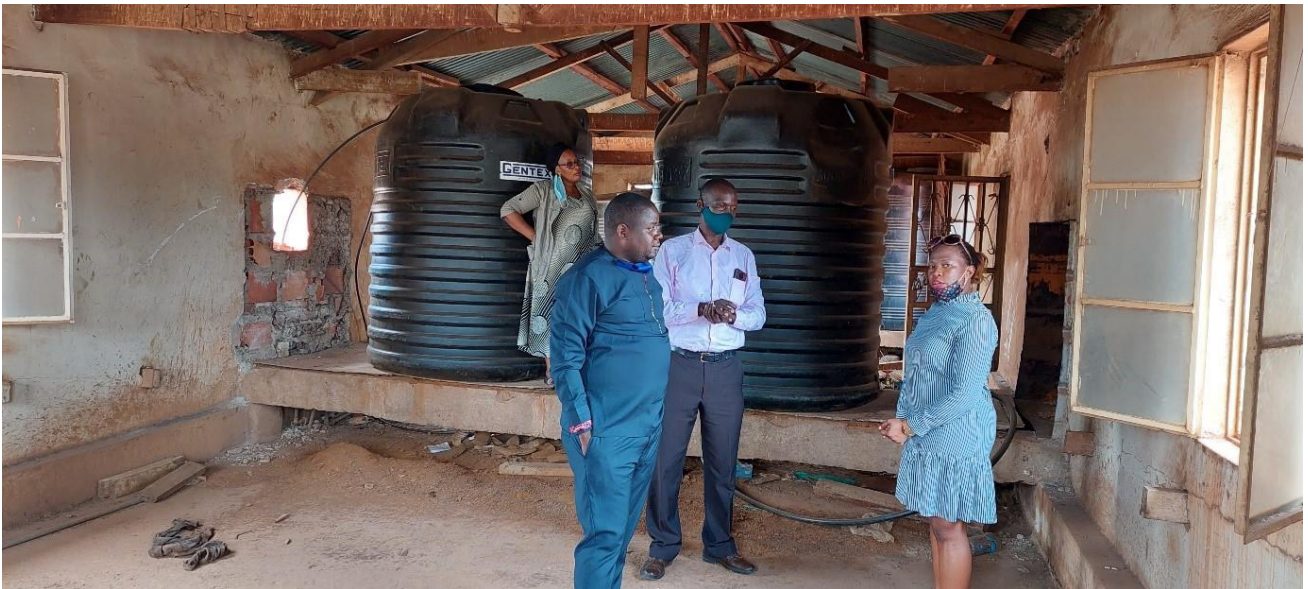
Figure 1; Some of the existing water tanks before upgrade.
