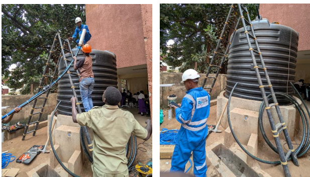
Figure 2; Photo of new tanks and solar pump installation by Davis & Shirliff
